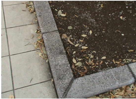
(a) roadside curb
