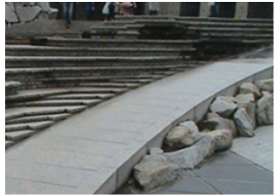
(b) slope road
