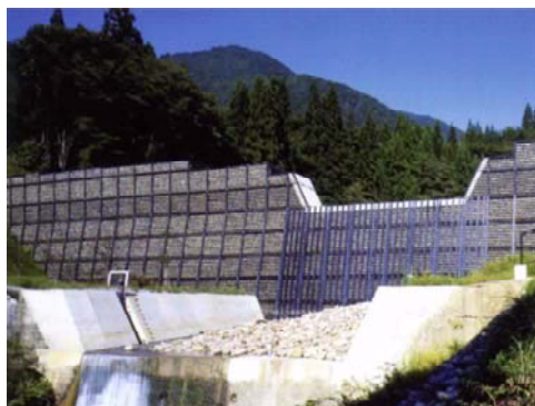
(a) 鋼製枠堰堤
